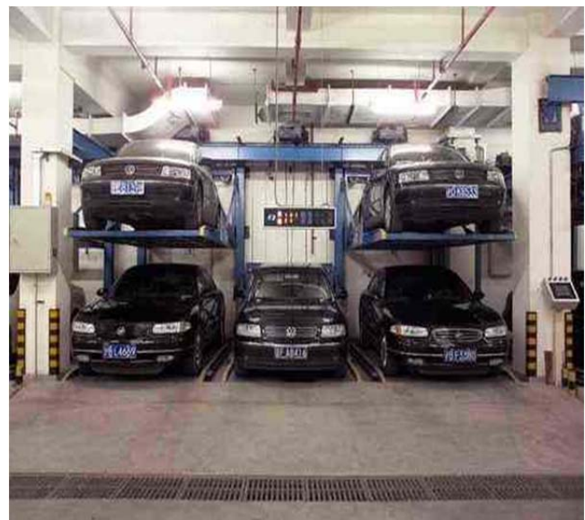
Fig. 12: Automated multistoried parking in basement underneath the piazza
